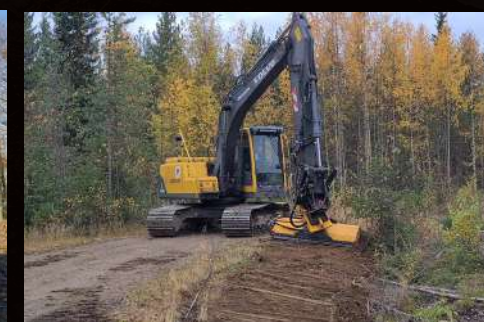
MC4-Hydraulic mounted to excavator
