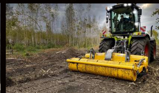
MJHS in land clearing
